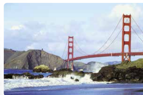
Golden Gate Bridge
